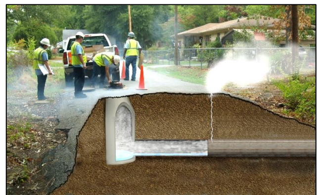
Photo Rendering of smoke testing: City of Brandon Mississippi.
